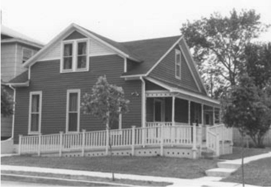
This home on Brown Street was recently renovated.
