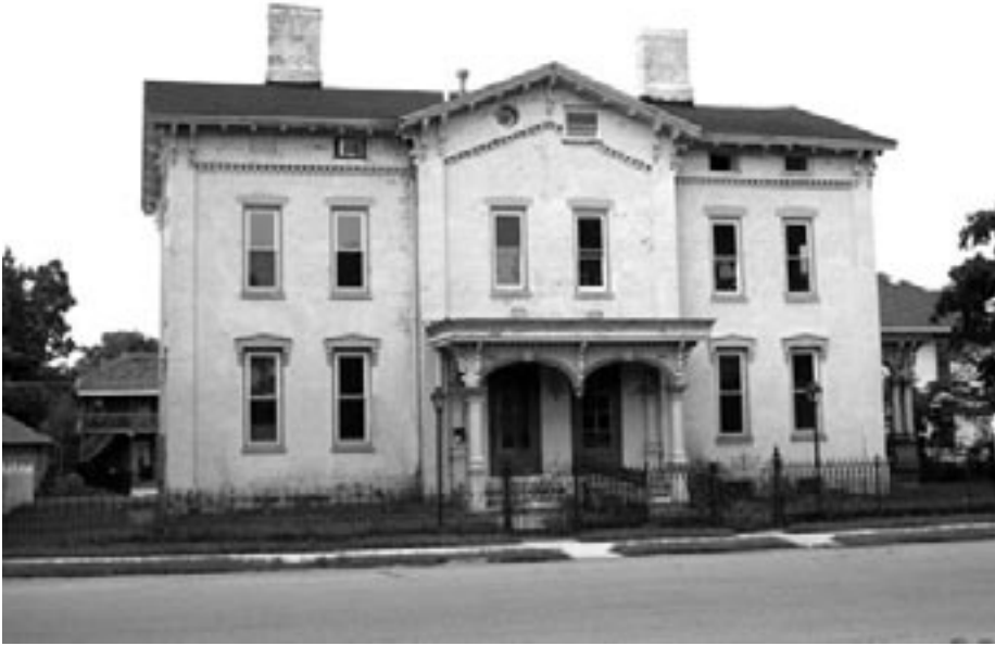
The John Levering House was built around 1850; it is located on Tippecanoe Street.
